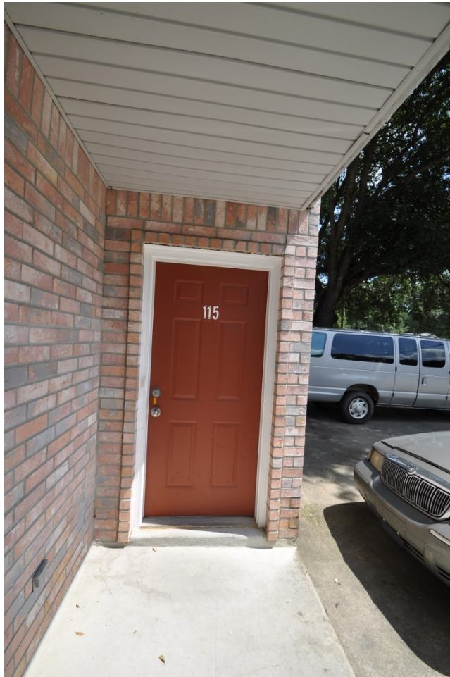
Downstairs flat at 700 S. Curran Ave.
