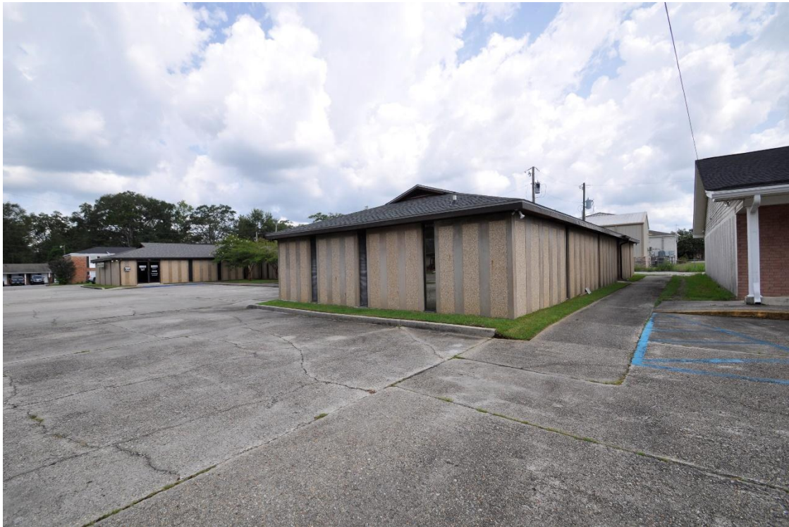
Right side of building
