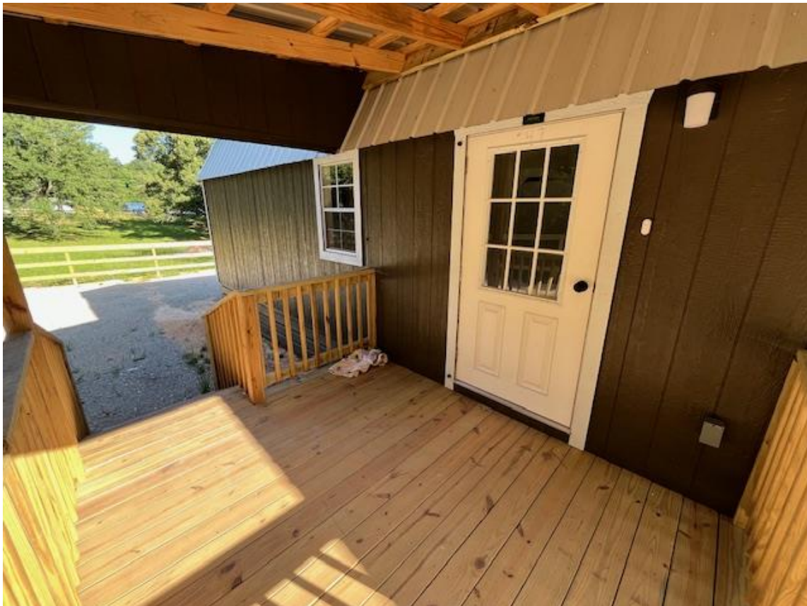
Covered front porch
